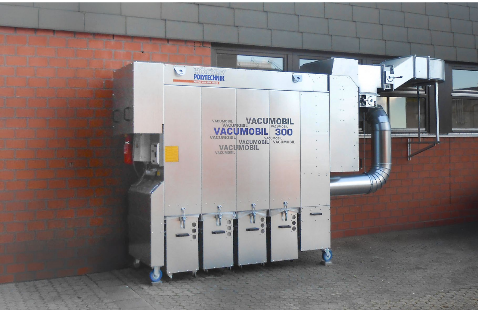
Vacumobil JT 300 used in wood processing, installed outdoors with return air and chip discharge into collection bins.
