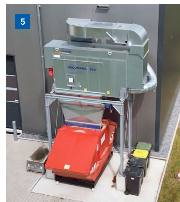
4 Vacumobil 350 with weatherproof enclosure for briquette press operation
