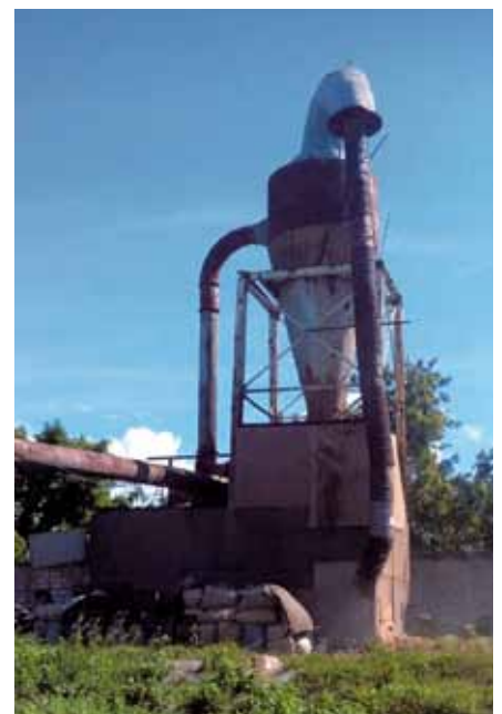
Before modernization – inefficient chip cyclone 75kW
