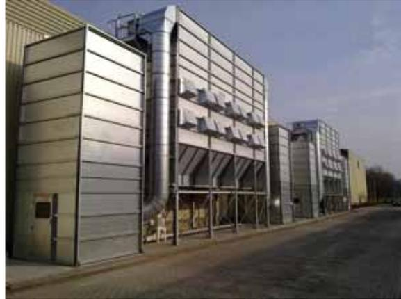
for this area alone. Another challenge was to use only one chip conveying system to transport the chips from the three new filter units to a final chip storage location. Höcker Polytechnik chose a high-pressure material transport blower with only **30 kW** of drive power. The high-pressure feed pipe with a total length of **300 metres** was also included in the scope of delivery.
